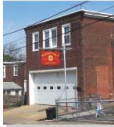
Independent Fire Company is located one block away from Pioneer.
