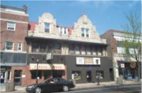
Inconsistent facade and streetscaping treatments detract from Uptown's historic charm.
