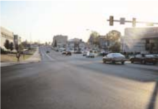
Large curb radii create a long pedestrian crossing at the intersection of Old York and Washington.
